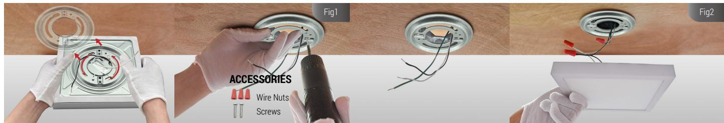
3. Use the CCT switch to select the desired light color. Arrange the wires into the J-box. Align the two rivets on the back of the light fixture with the holes on the wider side of the mounting plate, and then tighten them clockwise until the fixture is secure and parallel to the ceiling. See Fig3, Fig 4.
